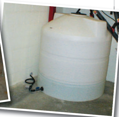
» Left: THE OVERALL VIEW of the fertigation system, controller and connections. » Middle: THE MODEL L 1000 INJECTOR PUMP in the pump room for the complex. » Right: THE 300-GALLON TANK in shop area, with the hose connection through the wall to the injector. The shop area was selected since it has easy access for the fertilizer delivery.
